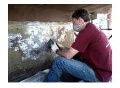
You definitely want to wear a mask and safety glasses for this because the grinder kicks up a lot of dust that can get in your face. A good grinder will have no trouble sinking in and removing the materials the keel is made from. Carefully work the grinder with a light touch pulling it towards you, as this gives you the greatest amount of control. Pushing the grinder away or from side to side tends to allow the grinder to bite into the keel generating deeper gouges than you really want to make.
